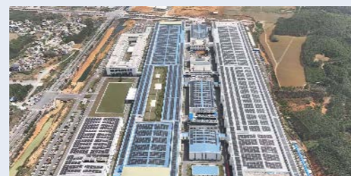
Photovoltaic Panels Installed on Rooftops in the Factory Area
